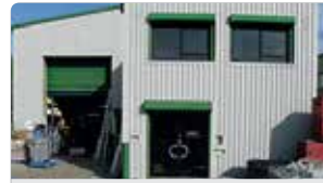
Coulson office expansion
