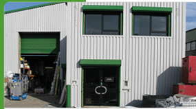
Coudsdon office expansion
